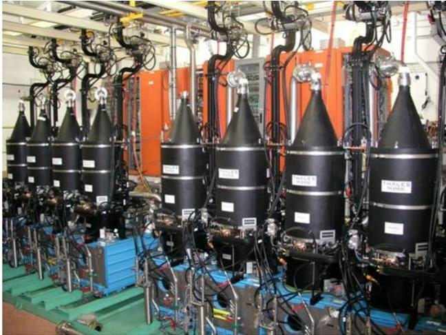
**Figure 1.10:** Tore Supra/WEST 700 kW/CW klystrons
