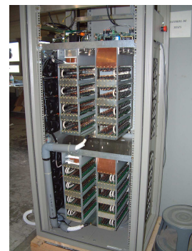
Fig. 6 High voltage inverter for plasma application
