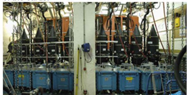
**Fig. 8:** Implementation of the protection opening switches (in the blue enclosures)
