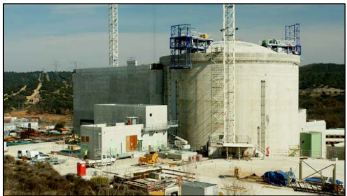
Early 2015: View of Reactor and Auxiliary Unit Buildings © CEA
