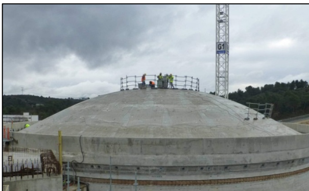
January 2015: Reactor dome concrete poured © CEA
