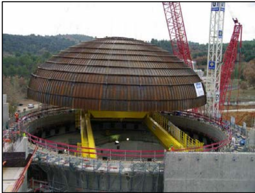
December 2013: Reactor dome installation © CEA
