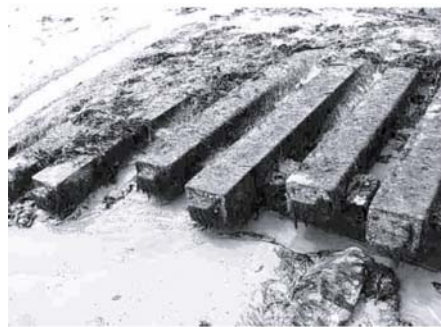
Figure 1. Prestressed beams during long-term exposure in marine environment
