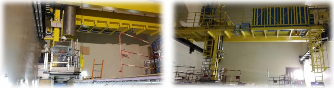
Fig. 6: One-site pool crane commissioning tests
