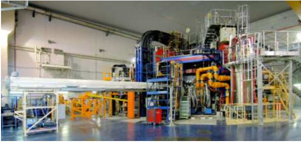
Fig. 1 - AIA connected to WEST Tokamak
