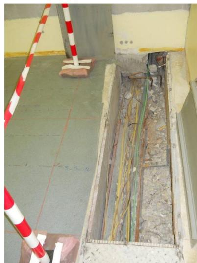
Figure 12: (left) Example of a CoMo measurement apparatus for contamination measurement, equipped with a plastic scintillator and Zns for the detection of  $\alpha$  and  $\beta$  particles and gamma rays, (right) Example of a duct to be checked, containing debris and cables.
